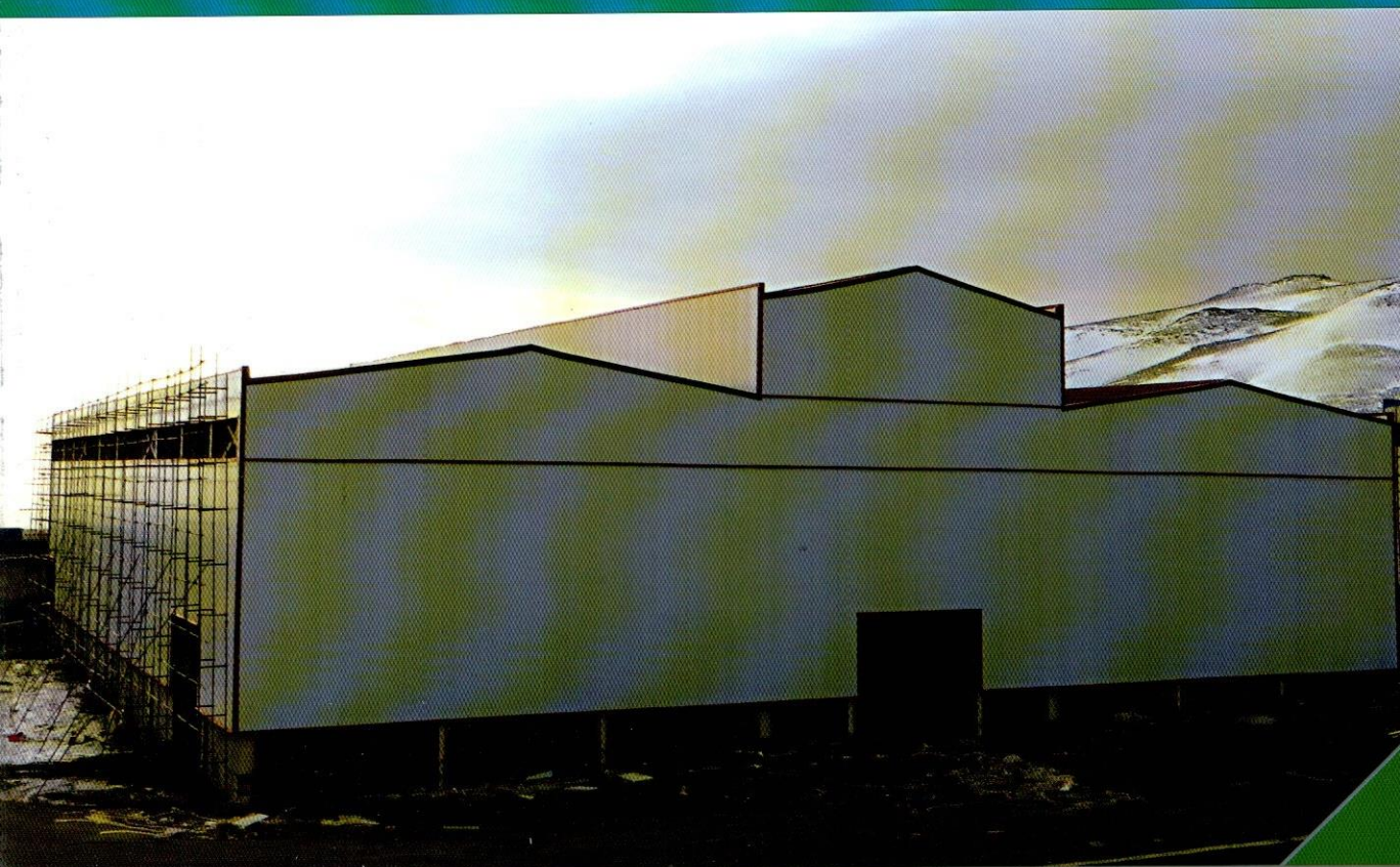
Roof of dairy center in Cremona
